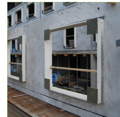
Spouwankers (geleverd door Hakron-Terwa) in prefab spouwblad.
